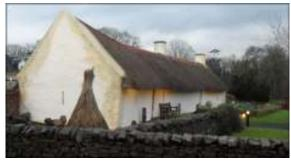
"The north-west gable is starting to crack, letting the wind and rain in and damaging the interior plasterwork."
