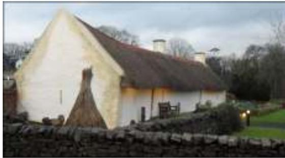
The trust has a plan to repair the cottage in stages. A wall at the end of the cottage will be propped up and pulled back in line with the rest of the building. Cracks along the walls and windows will be filled, and the roof rethatched and the outer walls re-limewashed, weatherproofing the cottage.
